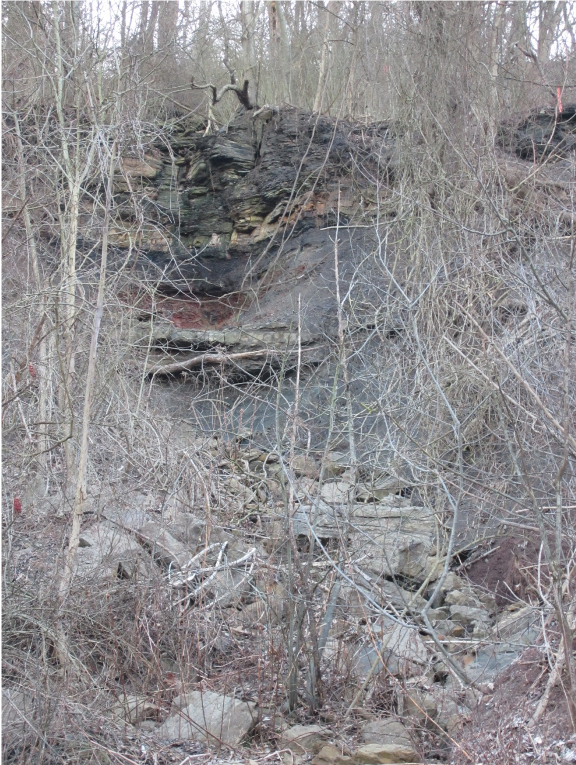
Closer view northeast at the eroded ravine at Sta 976.
