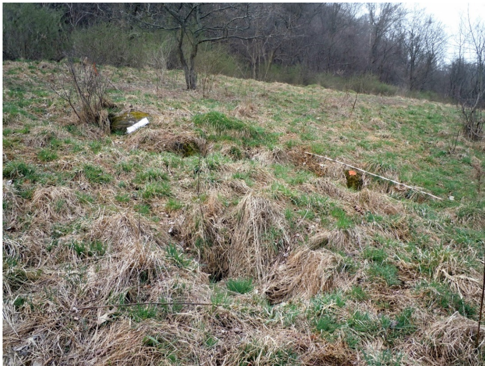
View southeast at the above cracks. Clipboard and 6 foot rule for scale.
