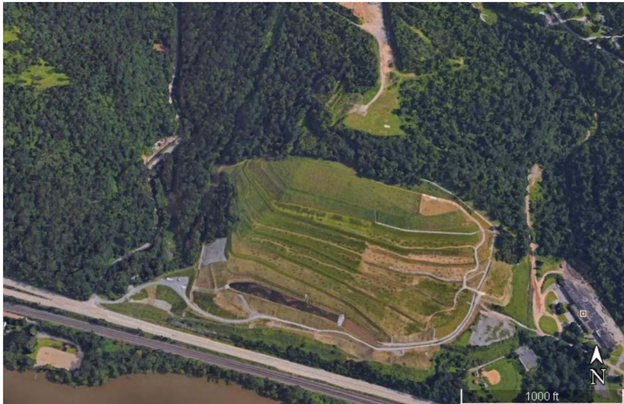
Figure 13. Google Earth photo of the restored Kilbuck Landslide site.
