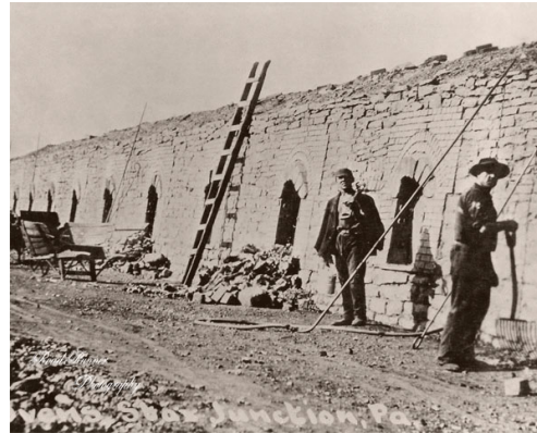
Figure 21. Bee hive coke ovens operated in Star Junction. The coke ovens were in Stickel Hollow on the Washington Run Railroad, which later was owned by the P&LE Railroad. It appears that the rail bed became the 4 lane PA 51. From Allison PA, 2013.
