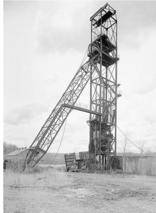
Figure 51. The tippie at the Maryland Shaft #2 of the Wilmore Coal Company at Wilmore. The shaft was about 850 feet deep.
