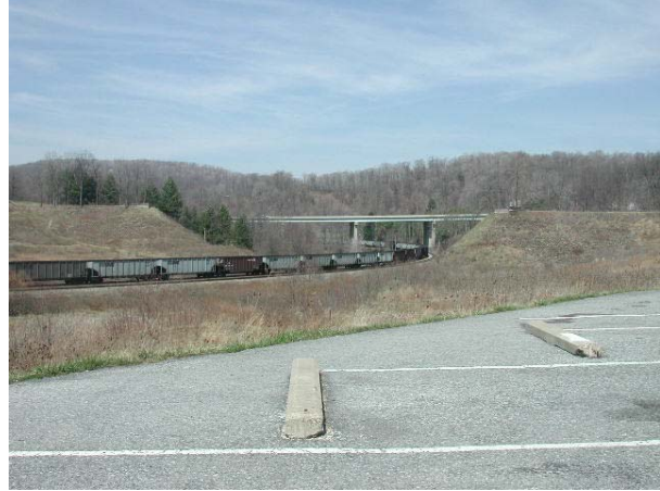
Figure 54. Photograph of the breached South Fork Dam as it appears today.
