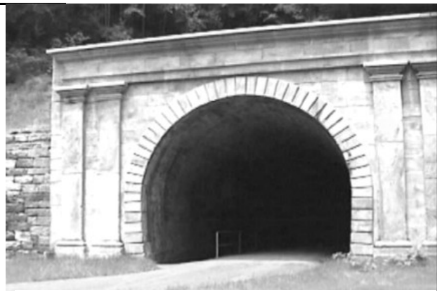
Figure 14. Photograph of the northeastern portal of the Staple Bend Tunnel. Photo by Kennedy (2001).
