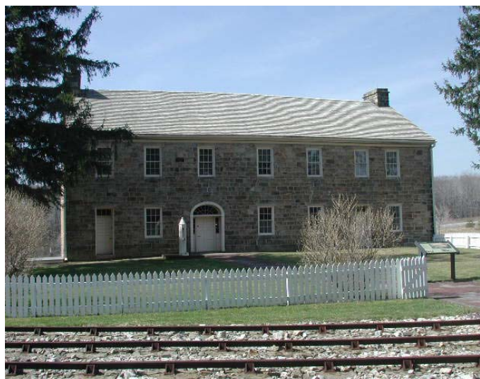
Figure 40. Photograph of the restored Lemon House at the Allegheny Portage Railroad National Historic Site.
