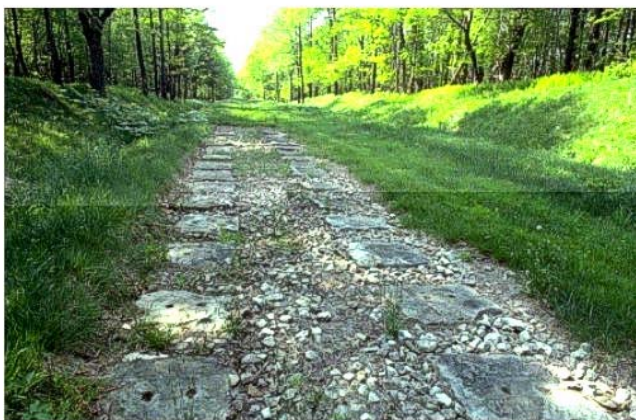
Figure 3. Photograph of stone “sleepers” along the Allegheny Portage Railroad right-of-way at the Allegheny Portage Railroad National Historical Site.
