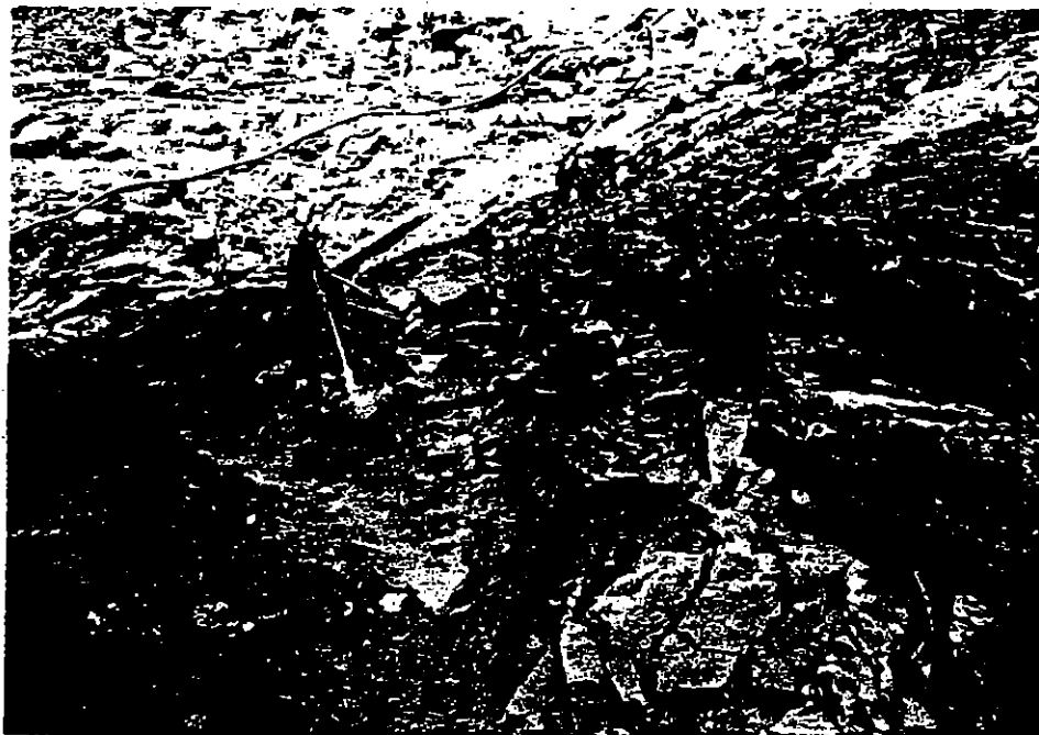
FIGURE 7 - HOSING JOINTS IN CORE AREA
