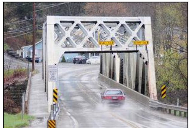
Bridge over Slippery Rock Creek in Wurtemberg
