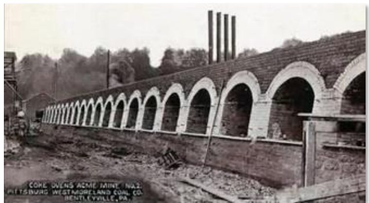
Historical photo of coke ovens at the Acme mines of the Pittsburgh-Westmoreland Coal Co. in Bentleyville, PA.
