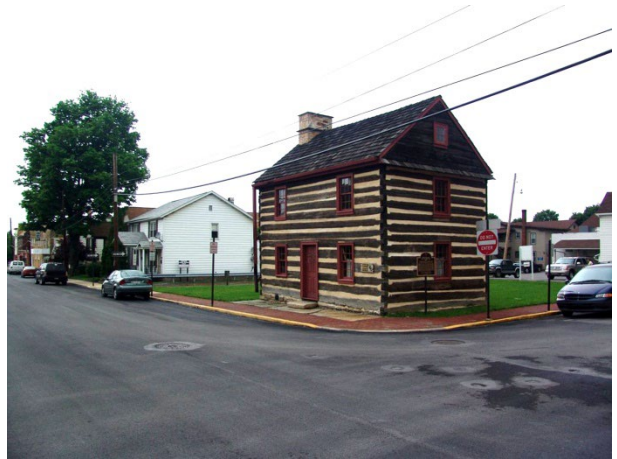
The historic Simler House, built around 1807 in Philipsburg, PA, was constructed by a Revolutionary War veteran named John Henry Simler. Over the years, it served as Simler’s home, a shoe repair shop, a school, a bakery and a tavern.
